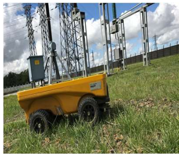
HIGHT VOLTAGE TRANSFORMERS
