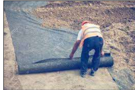
Geotextile laying
